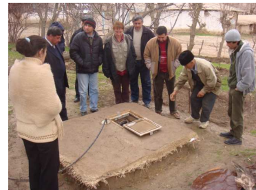
Completed water harvesting pond supplied with rainwater from nearby rooftop
