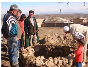
Re-confirming the exact dimension of the rainwater harvesting structure under construction
