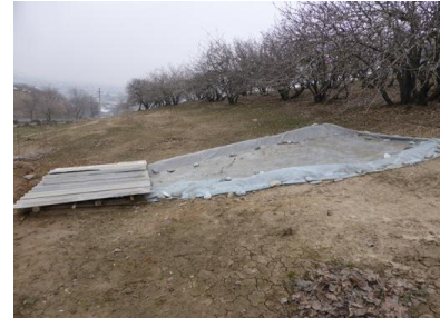
Concrete reservoir covered by roofing sheets, fed by a plastic-lined rainwater collection area
