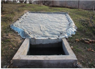
Concrete reservoir with plastic sheet for rainwater collection
