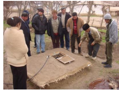
Completed water harvesting pond supplied with rainwater from a nearby rooftop
