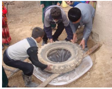
Placement of a car tire on top of a water storage pond through which water intake and outtake is processed
