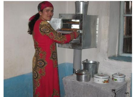
The “6 in 1 *heat exchanger*” (see above photo on the right site) allows rural families to engage in room heating, cooking, tea preparation, warming up of water for washing and bathing- all at once.
